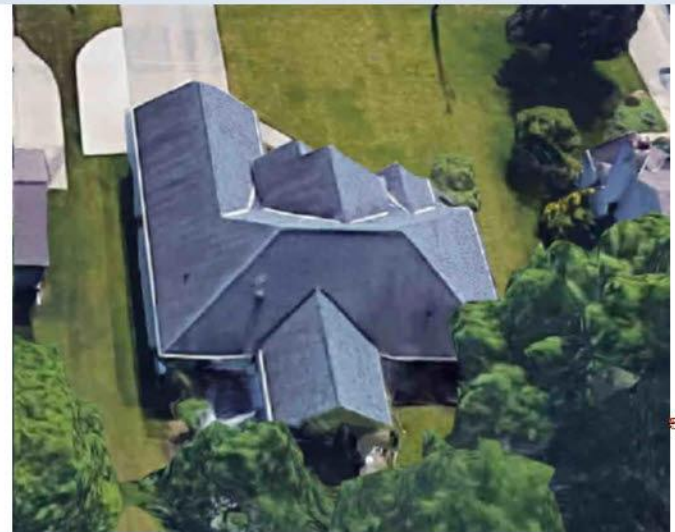
West Side View
