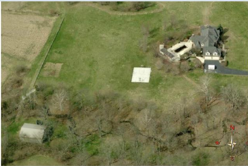
North Side View
